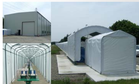
Superconducting Conductor Jacketing Building
