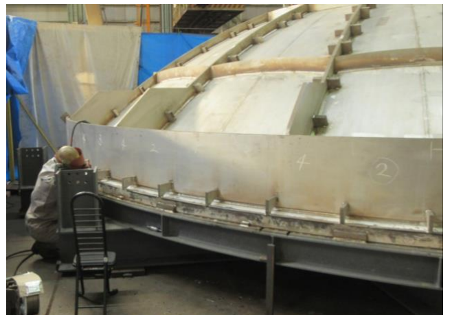
Figure 2: Reinforcing ribs and stiffening rings being installed
