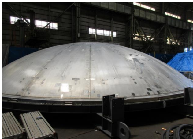
Figure 1: Nine sectors welded
