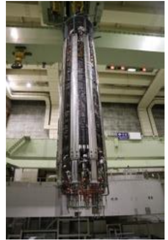
Central solenoid lifted
