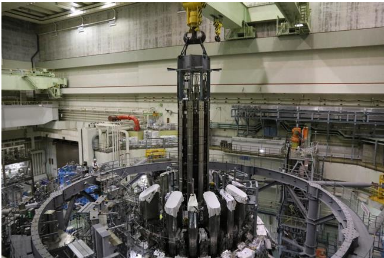
Insertion of central solenoid in the centre of the JT-60SA tokamak
