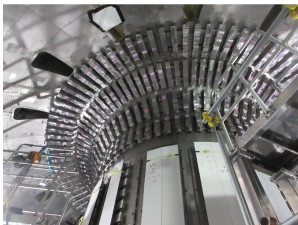
H-section steel supports installed in the upper divertor region
