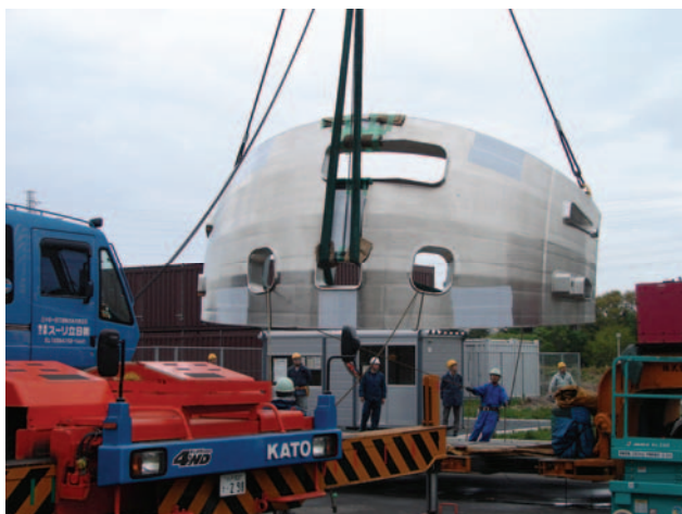
Outboard segment of 40° sector being unloaded at Naka
