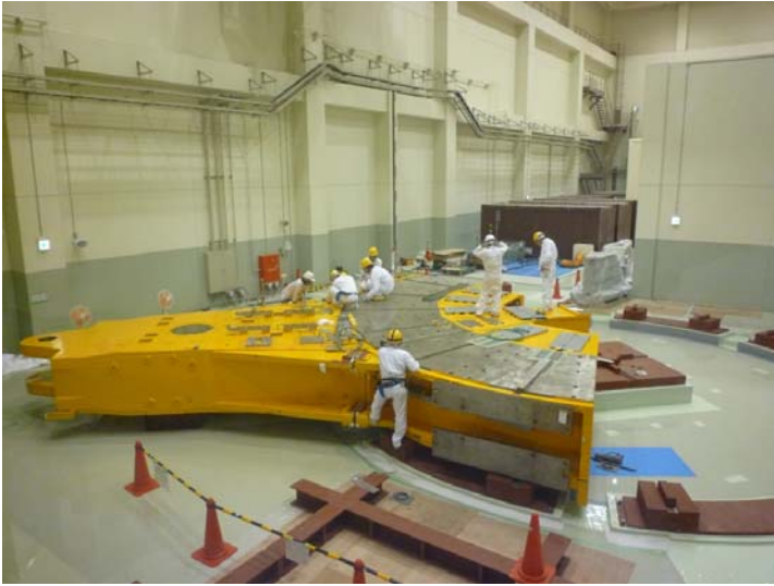
Disassembled upper support structure stored in storage building
