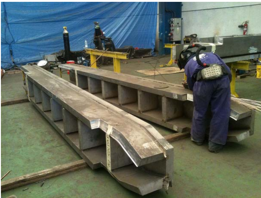
Welding of cryostat base radial legs
