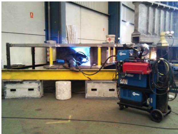
Figure 3: Welding of a double ring sector
