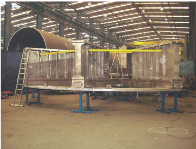
Figure 1: Dimensional inspection of lower structure sector
