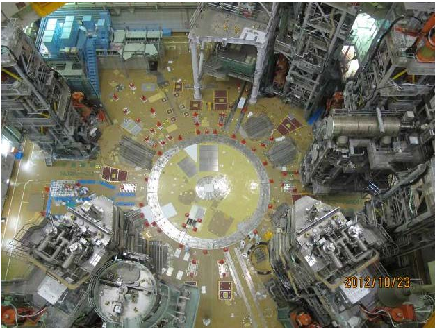
Torus hall after completion of disassembly
