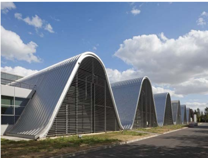
Figure 2: NEUROSPIN building at CEA Saclay
