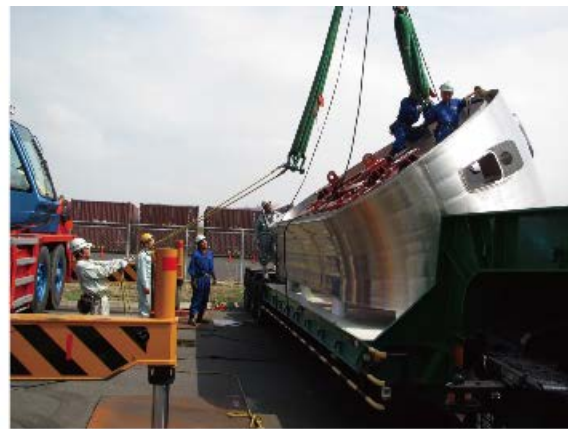
Figure 2: Loading sixth 40° sector onto a truck
