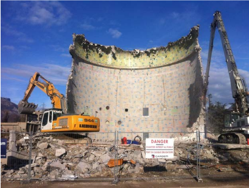
Figure 1: Demolition of the Siloe reactor building (February 2013)
