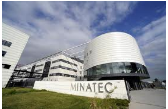
Figure 3: CEA Minatec Entrance
