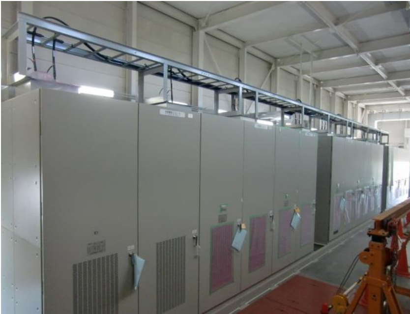
Figure 1: Power panel for inverter in the upgraded inverter building
