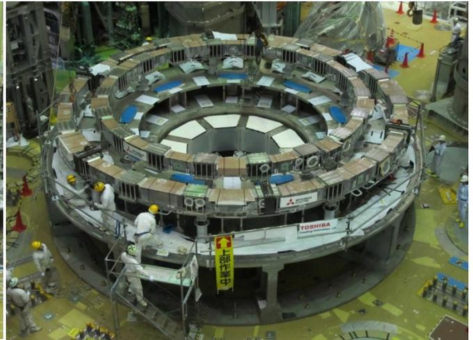
Figure 2: Coils temporarily installed on the cryostat base
