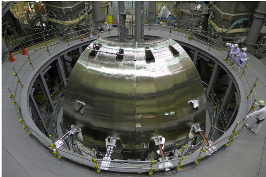
Figure 1: VV sectors (VV-D03 and VV-D04) installed on the cryostat base
