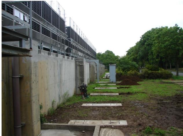
Figure 3: Support frame foundation for water supply pipes
