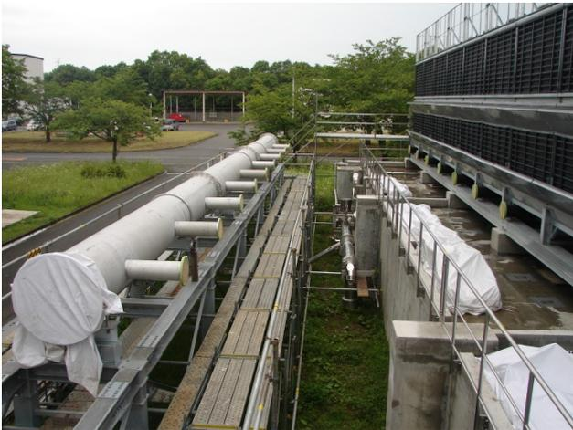
Figure 2: Installed water supply pipes for cooling tower
