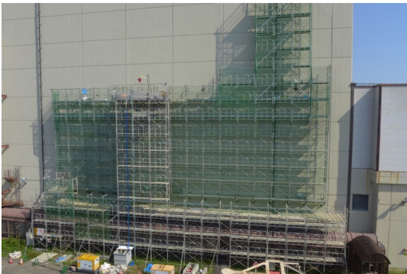
Figure 2: Scaffolding assembled on the JT-60 experimental building
