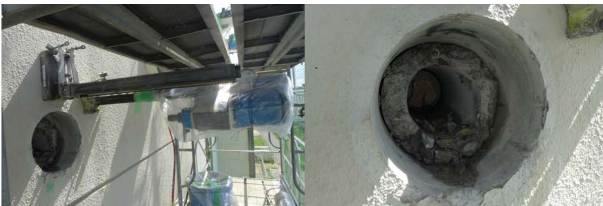
Figure 3: Open holes drilled by wet core drilling method
