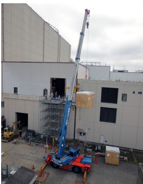
Lifting of QPC components up to the extension area of the JT-60 experimental building
