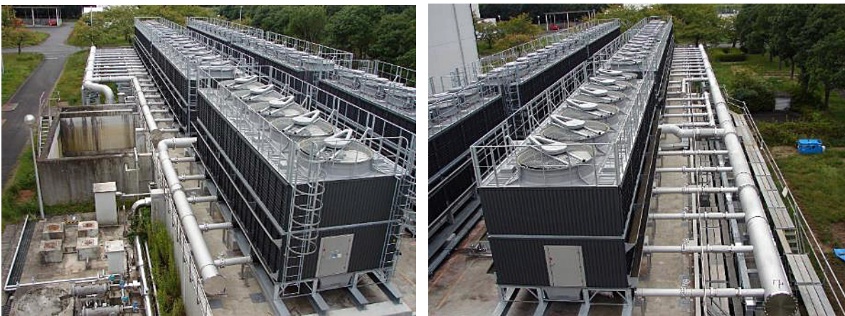
Installed pipes in the north (left) and south (right) of the secondary cooling system
