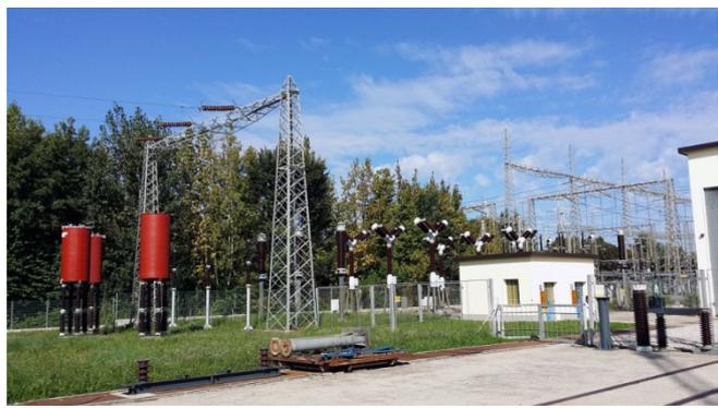
Figure 4: Detail of the SVEPPI switches and lines connected to the 220 kV substation
