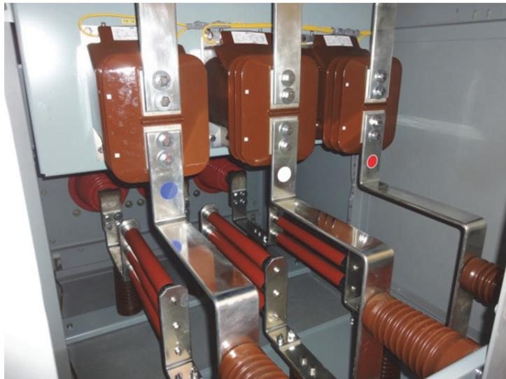
Figure 1: New resistors to suppress the current surge at the 18kV main AC power distribution line of the power distribution system
