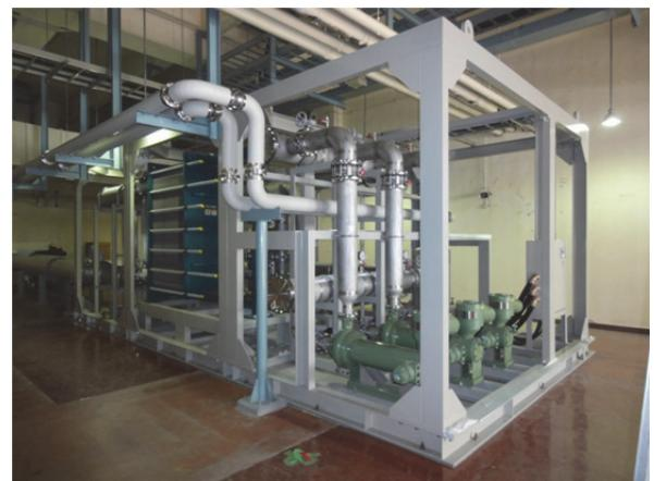
Figure 3: Demineralized water-cooling system for PF coil PSs
