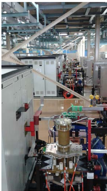
QPC installed in the rectifier room
