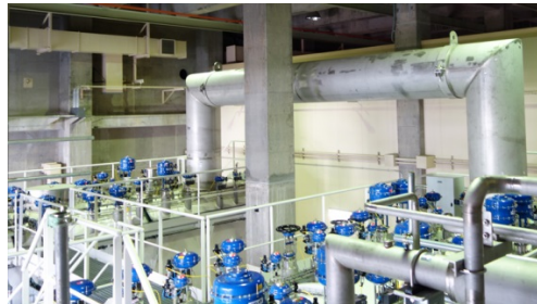
Figure 3: Top of the RCB and ACB connected by the cryogenic transfer line
