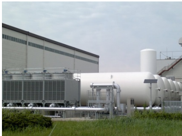
Figure 2: The high-voltage transformers and water cooling towers, gaseous helium storage vessels, and liquid nitrogen tank (from front to back)
