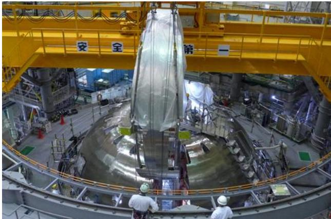
Figure 3: Inserting the final 20° sector temporarily
