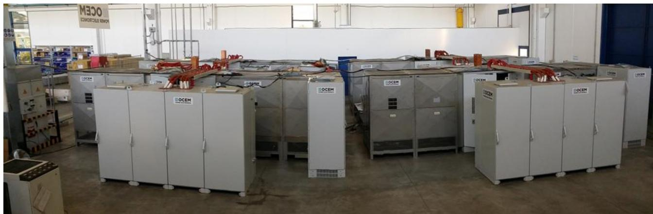
Figure 2: 4 SNUs and LCC installed in the OCEM premises reproducing the final installation at the JAEA Naka site.
