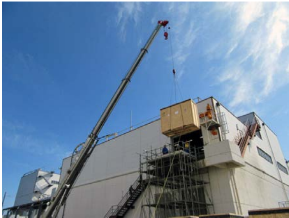
Figure 4: Lifting the EF PS boxes into the rectifier building
