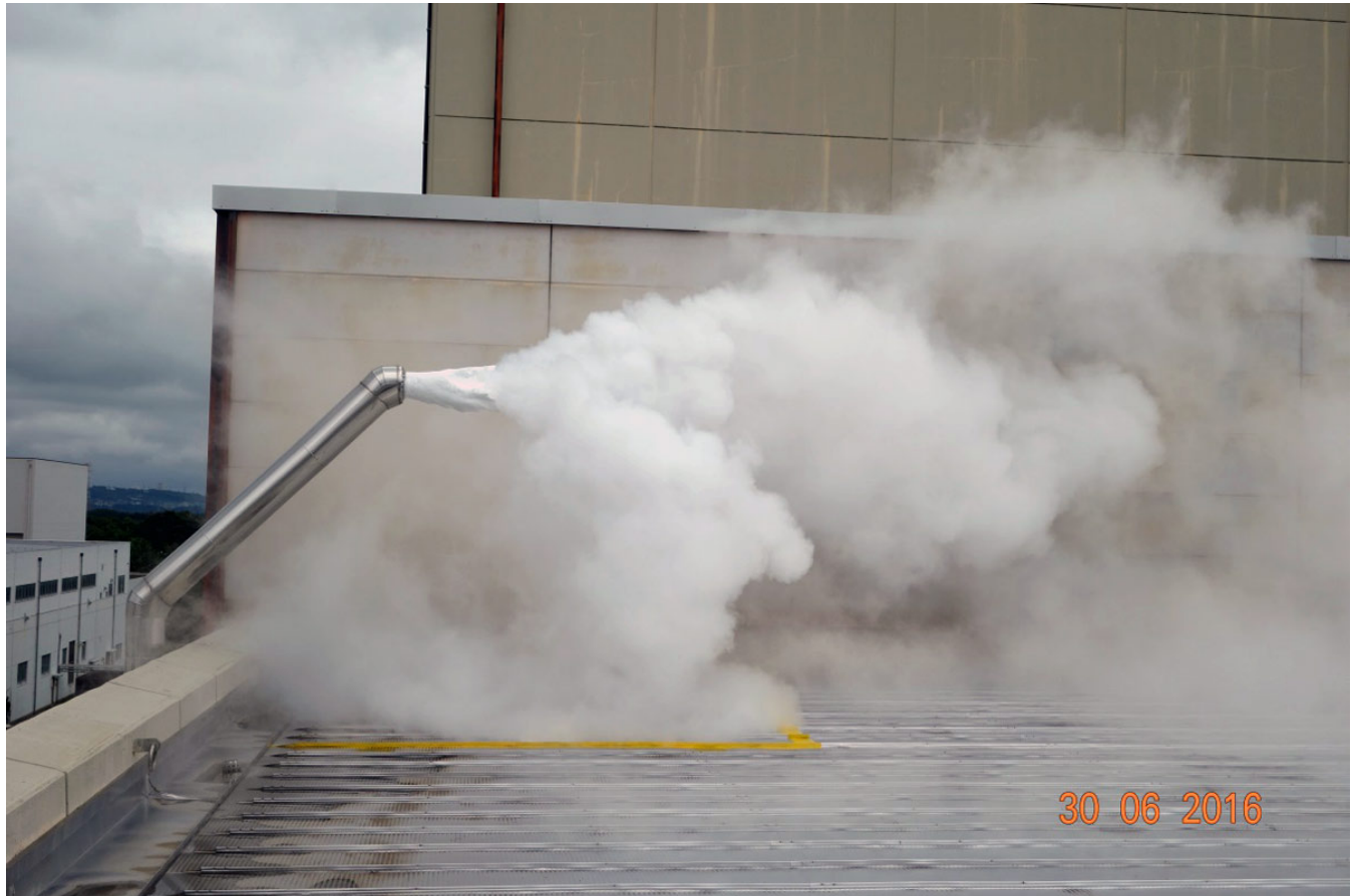
Figure 1: Venting of gaseous nitrogen above the cryogenic hall during the baking test
