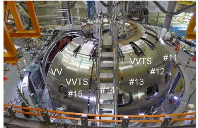
Figure 2: A total of 15 VVTS sectors has been mounted
