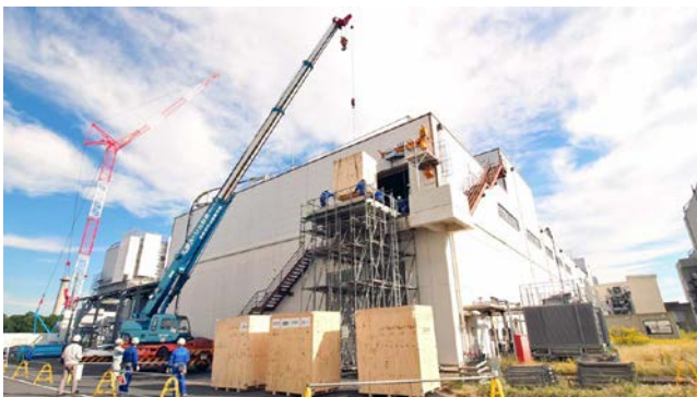
Figure 6: Lifting the SNU boxes into the rectifier building
