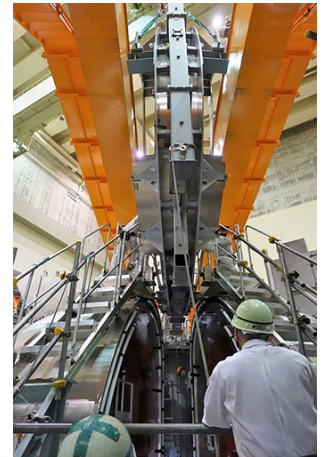
Figure 3: Inserting the final 20° sector
