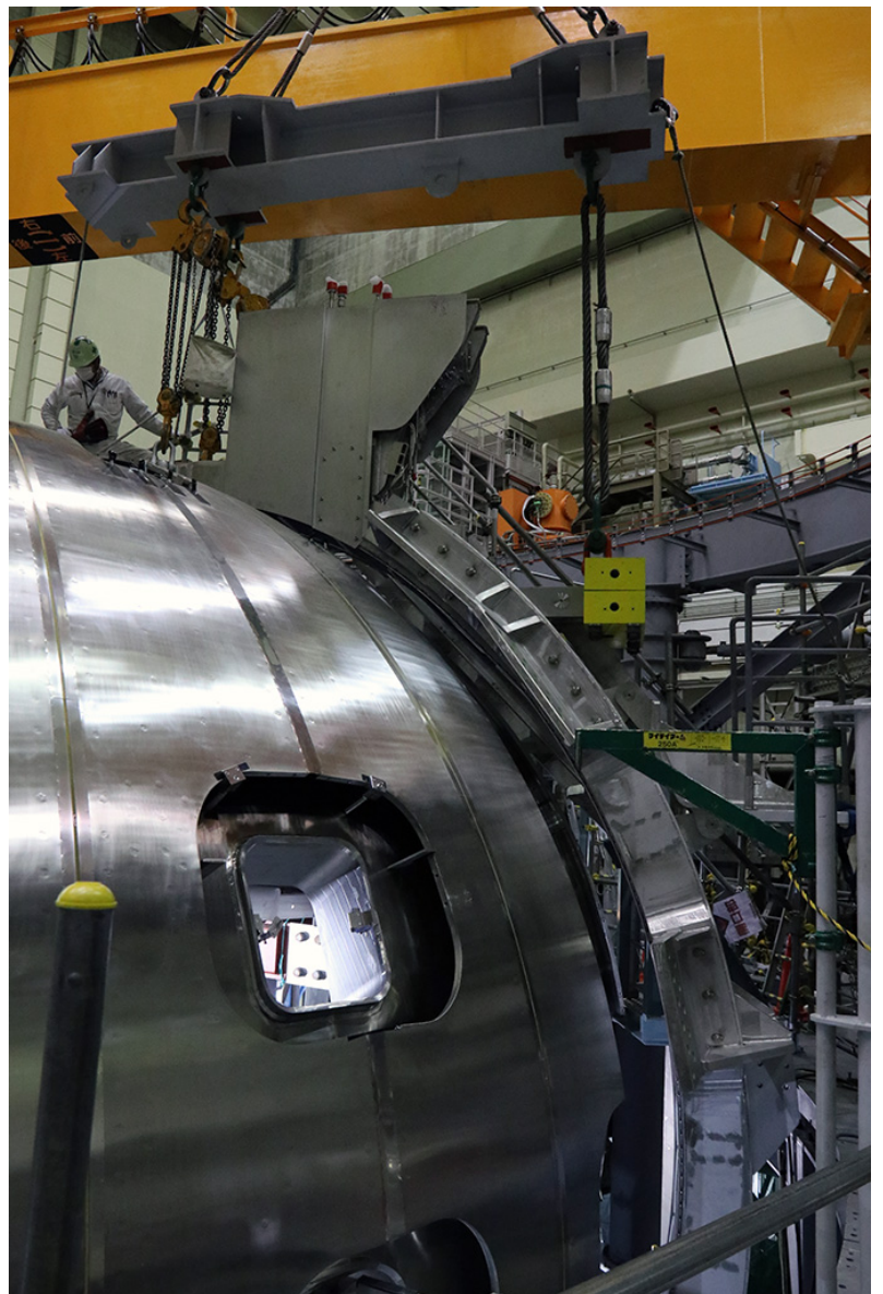
Figure 4: Mounting - "Sandra" - on the JT-60SA torus
