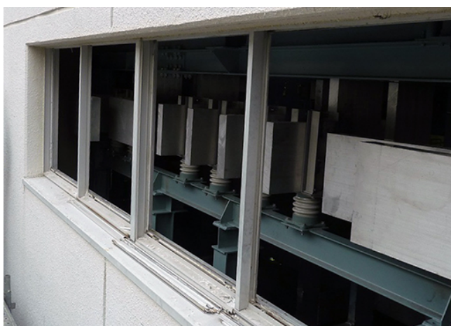
Figure 3: Existing windows to be used as feedthroughs
